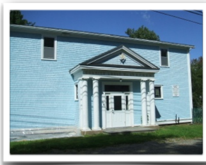
Exterior view; views to the East, West, North and South.
