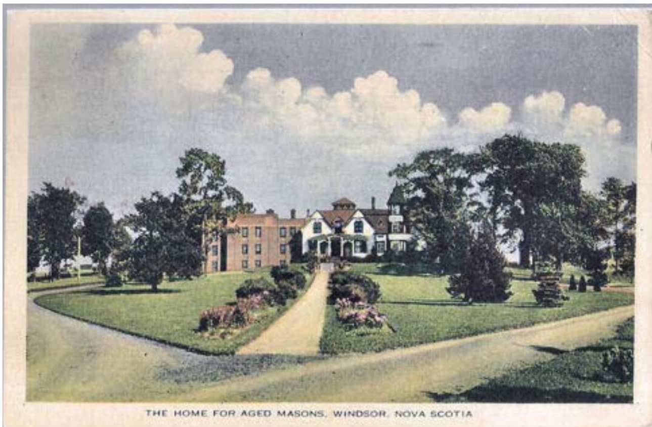
Picture of the former Nova Scotia Freemasons Home in Windsor, NS. Torn down after it was no longer able to meet the building code for nursing homes
